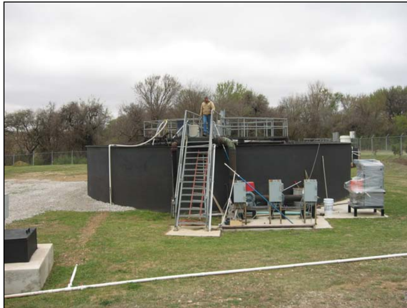
Figure 4.5: Rhome West WWTP – Concentric Circle Type WWTP
