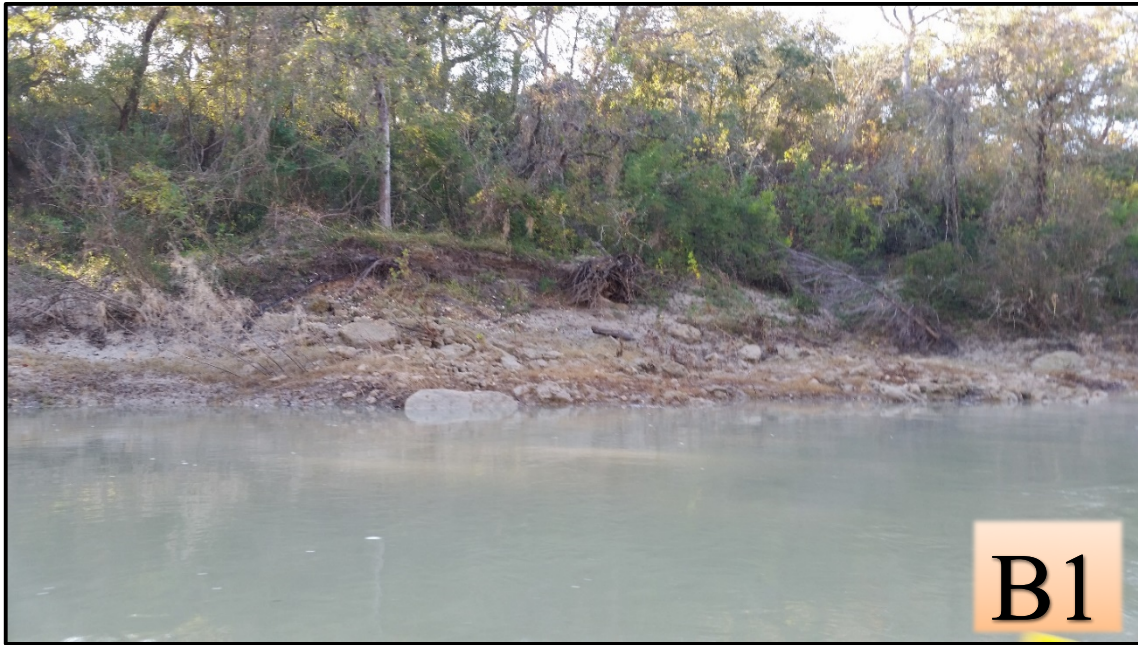
Figure 64. Location of B1. Photograph taken near Cuero, TX, (December 6, 2016).
