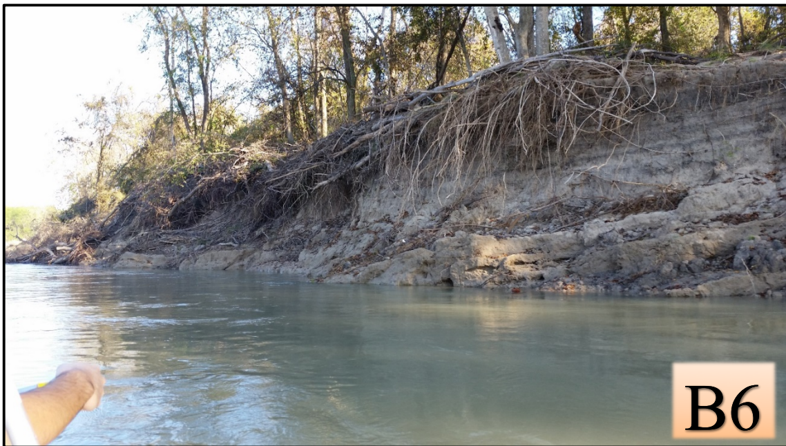
Figure 69. Location of B6. Photograph taken near Cuero, TX, (December 6, 2016).
