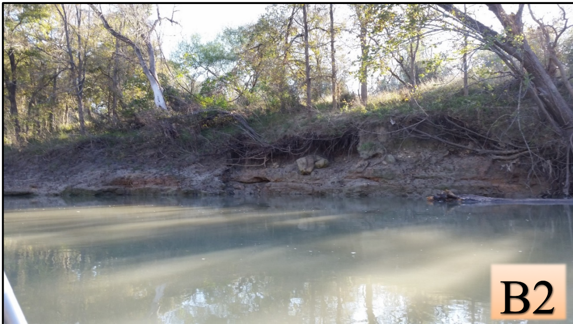
Figure 65. Location of B2. Photograph taken near Cuero, TX, (December 6, 2016).
