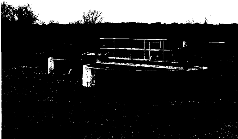
Figure A-7: Mixed liquor final clarifiers.
