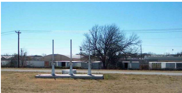
Figure 2-22 Gate Operators for Storm Drainage Sumps
