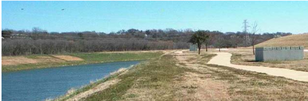
Figure 2-18 Sanitary Sewer Mains 248 (Foreground) And 1-I-1 (In The Distance) Siphon Crossings Of The West Fork Trinity River East Of North Main Street
