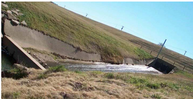
Figure 2-26 Storm Drainage Outfall TXR1
