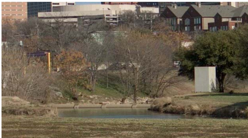
Figure 2-19 Sanitary Sewer Main 272-B Siphon Crossing of Inlet to the Clear Fork Trinity River, Located North of Forest Park Blvd.
