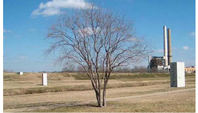
Figure 2-17 Sanitary Sewer Main 132 Siphon Crossing, (now abandoned), of The West Fork Trinity River Located North of The TXU Power Plant.
