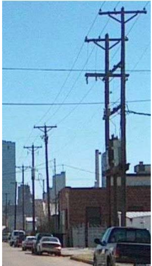
Figure 2-31 Overhead Power Lines
