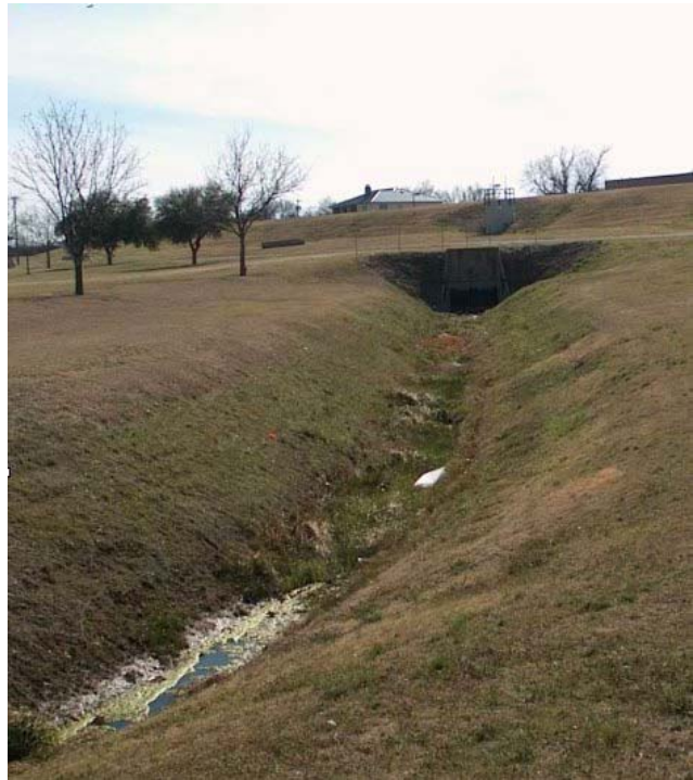
Figure 2-23 Storm Drainage Outfall MW1
