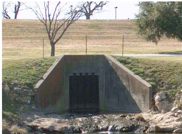
Figure 2-24 Storm Drainage Outfall MW2
