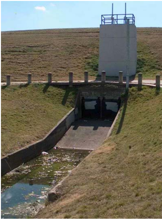
Figure 2-25 Storm Drainage Outfall SH1B
