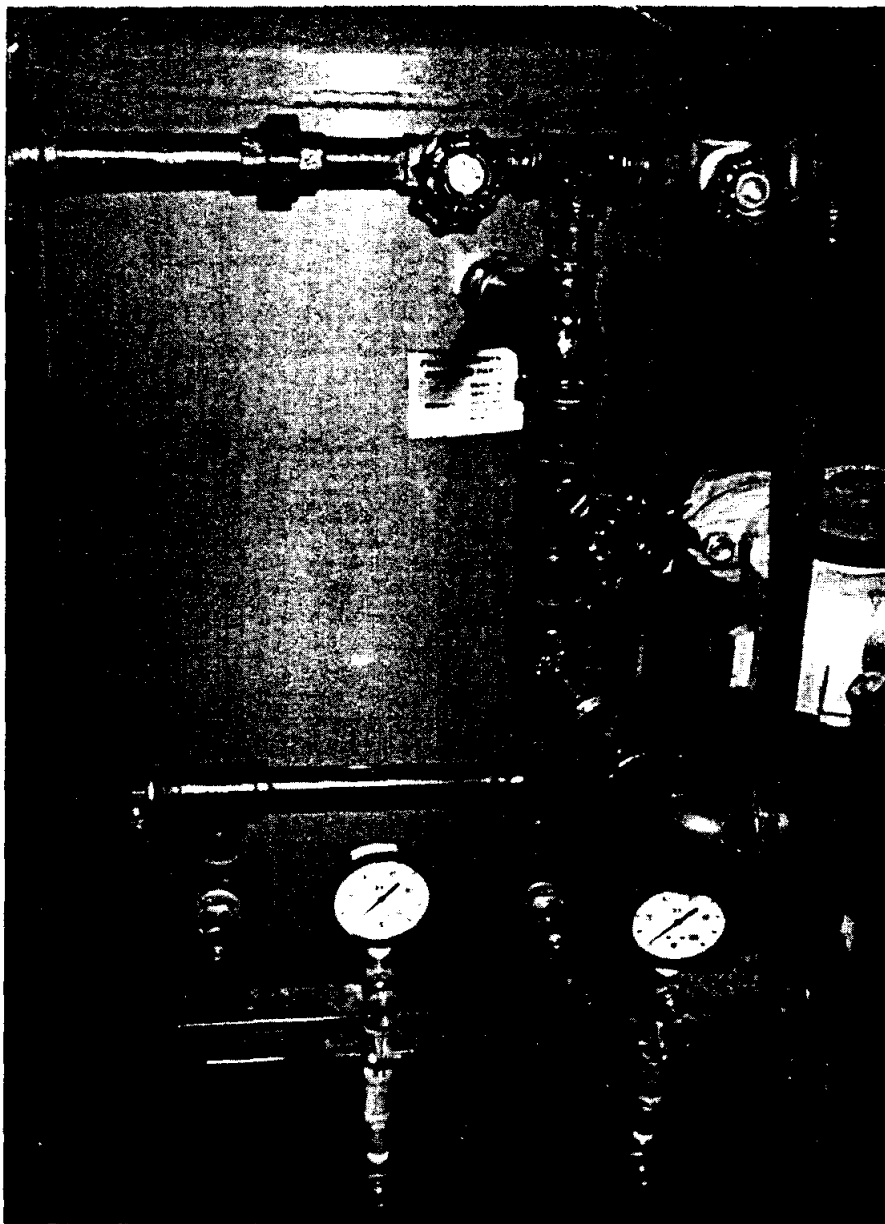
Regeneration water from the ion exchange process passes through the complexer tank before final disposal.
