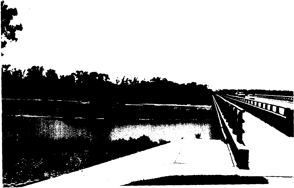
1-15 Island of sediment in channel at north Lake Houston Parkway bridge. View is downstream from north end of bridge.
