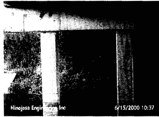
Figure 13: Beam-column connection
