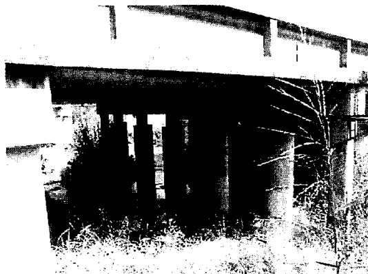
Figure 70: Bridge at Buss 77 Road
