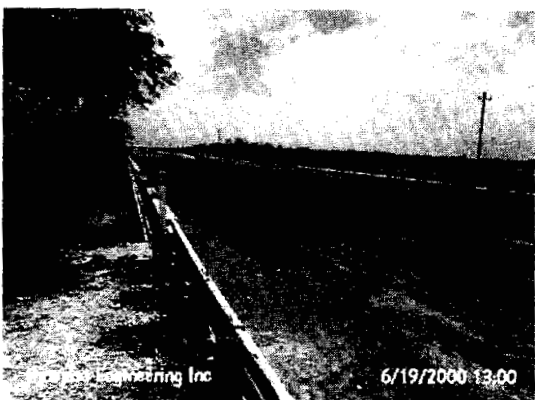
Figure 104: Bridge at FM 186
