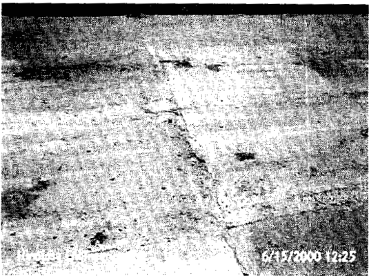
Figure 48: Cracked slab
