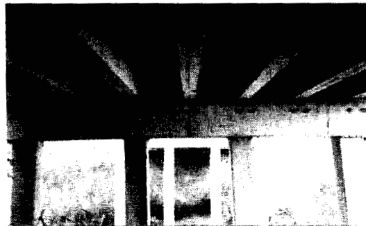
Figure 64: Double t-beam slab
