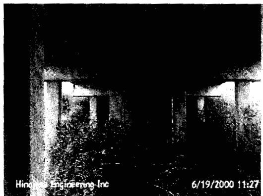
Figure 86: Double t-beam slab
