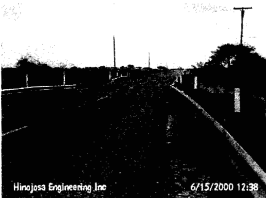
Figure 54: Bridge at FM 1761
