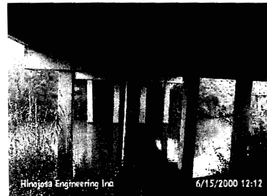
Figure 43: Double t-beam slab
