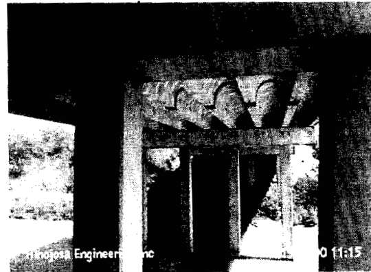
Figure 82: Double t-beam slab
