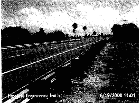
Figure 78: Bridge at 77 North
