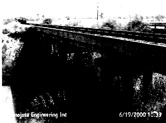
Figure 68: Bridge at Buss 77 RR
